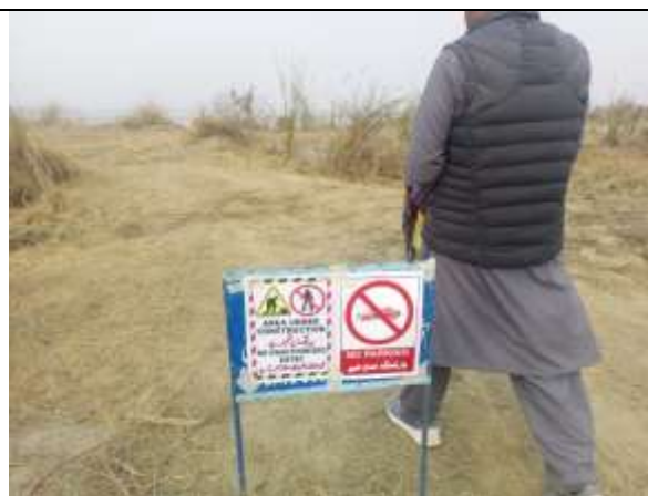
Sign boards Installed
