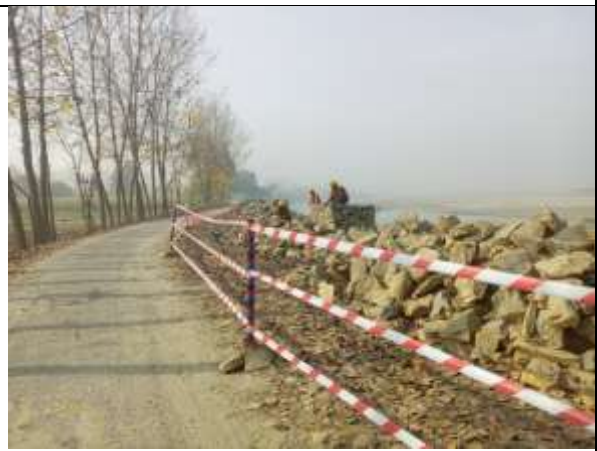
Proper Barricading done
