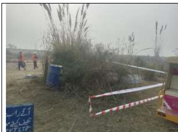
Proper Barricading of Site
