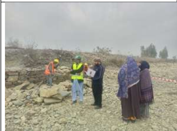
Barrication of Site
